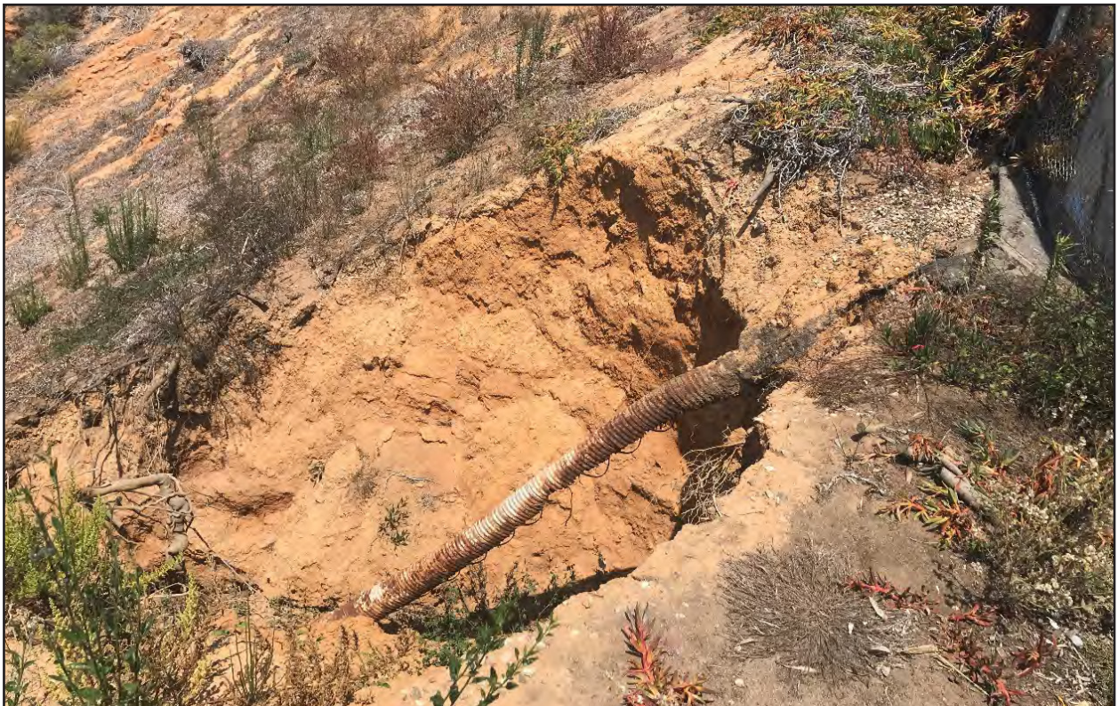
Slope Restoration Site 2
