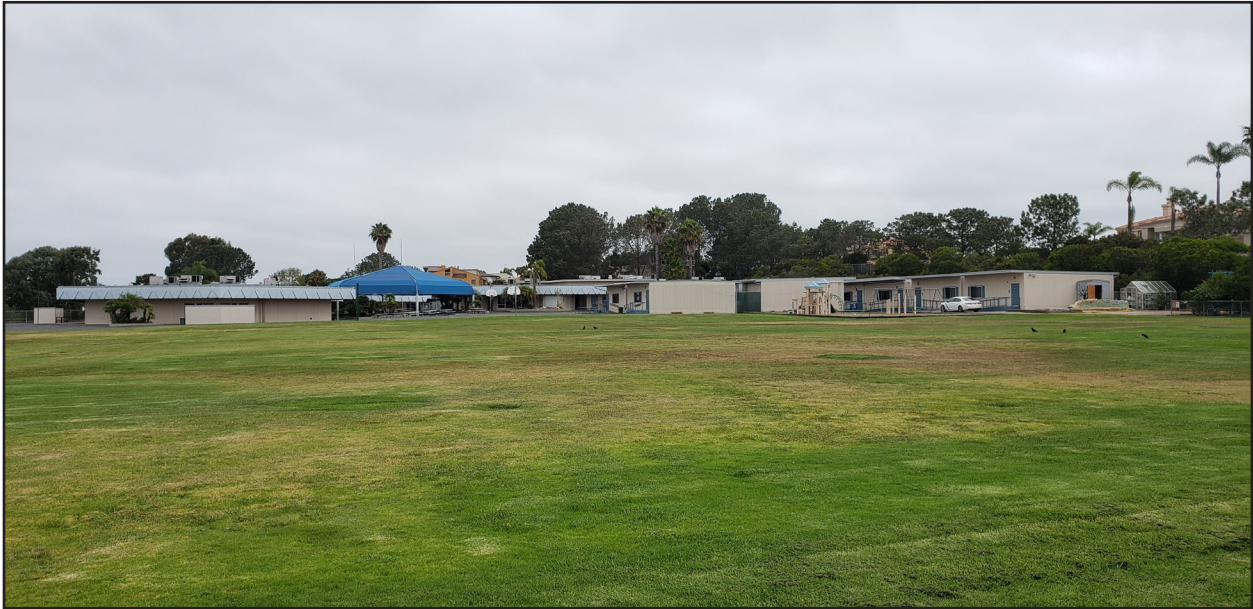
View from the play field looking north toward the school buildings.
