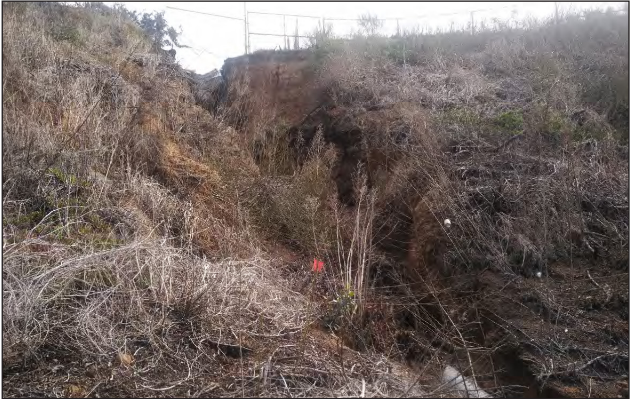
Slope Restoration Site 1
