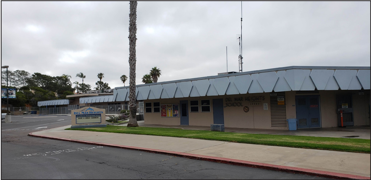
View of the project site looking southeast near the project driveway at Boquita Drive.
